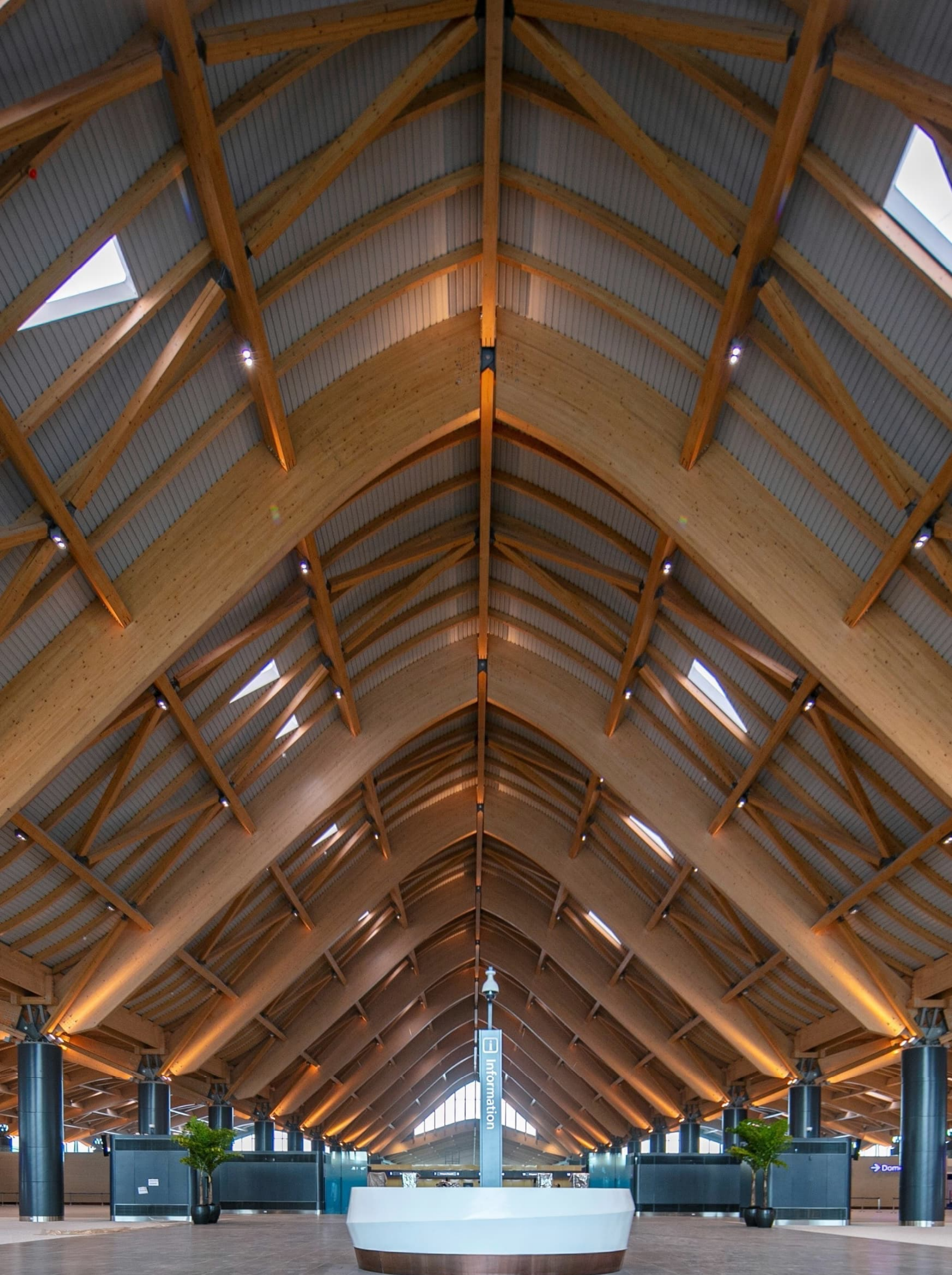
NOW OPEN: the long-anticipated new passenger terminal at the Clark International Airport (CRK), which was inaugurated by President Ferdinand Romualdez Marcos, Jr. on September 28, 2022.
